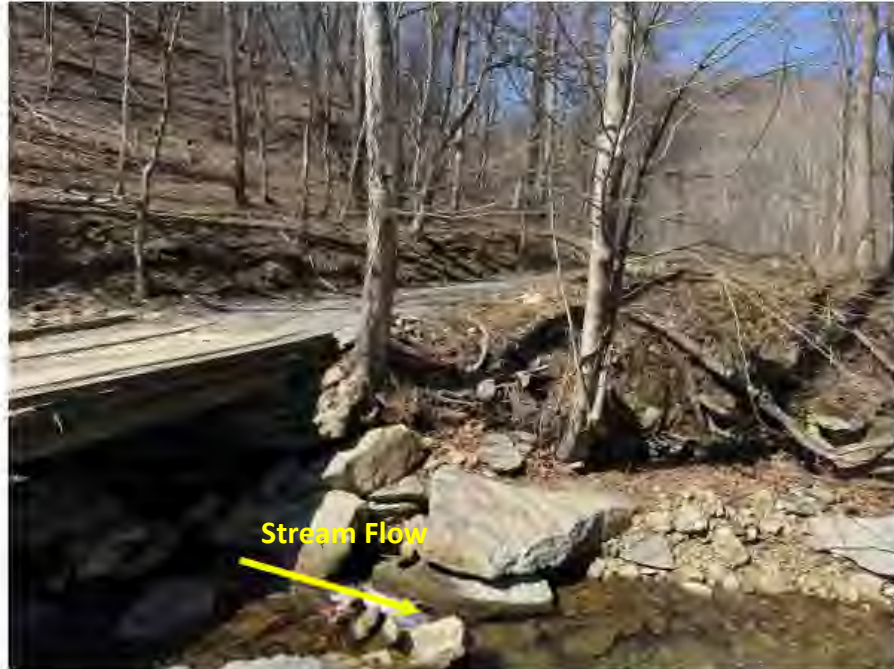
Photograph No. 1: View looking North
