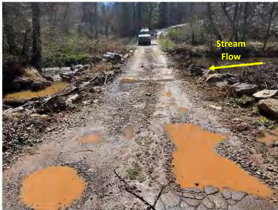
Photograph No. 2: View looking South
