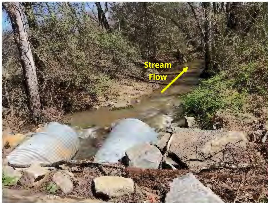
Photograph No. 4: View looking downstream
