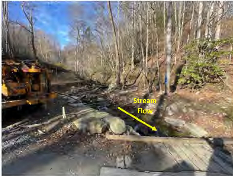
Photograph No. 3: View looking upstream
