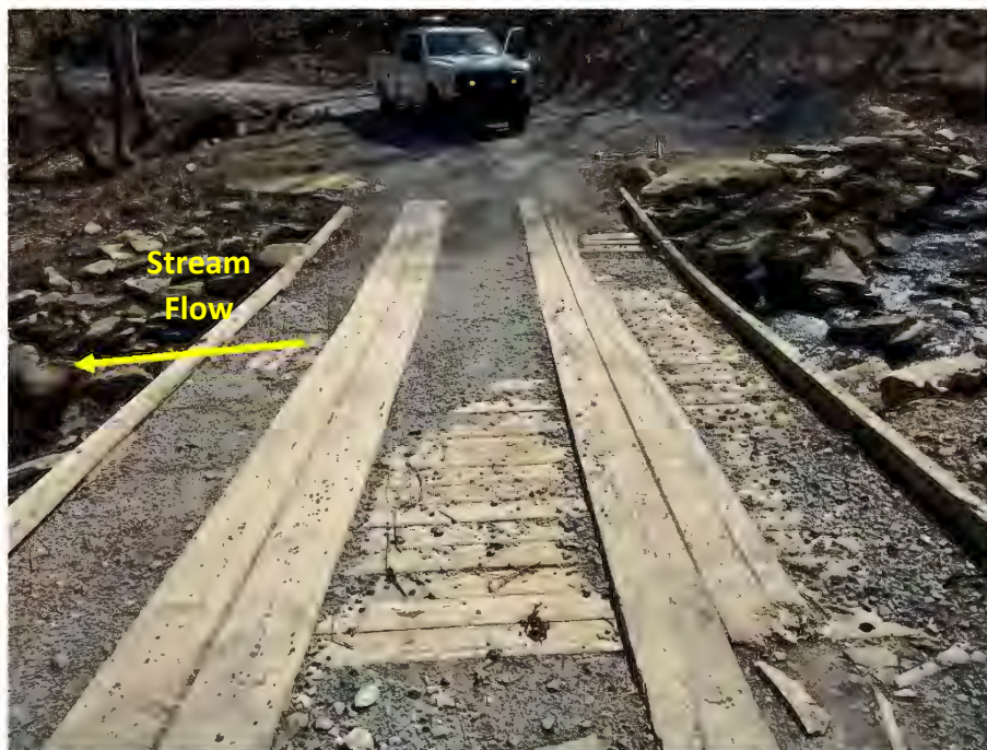
Photograph No. 2: View looking South
