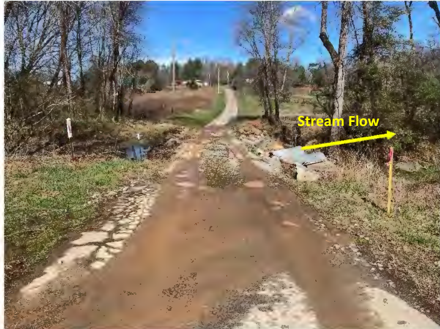
Photograph No. 1: View looking North
